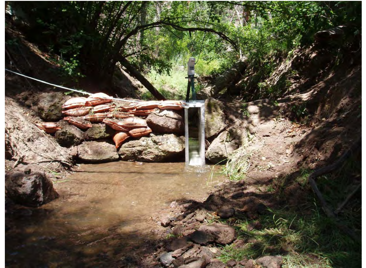
Figure B-2 Photograph of gaging station D123.6, a portable Parshall flume, looking upstream
