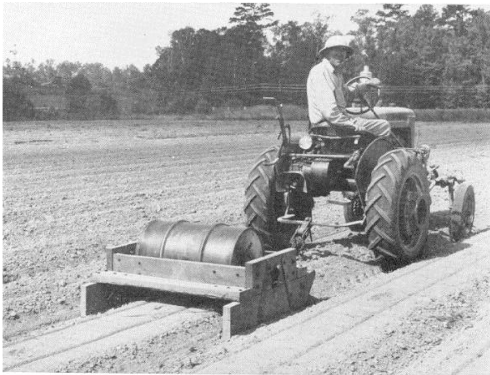
FIGURE 16.—A 1-row roller constructed in a farm shop.
