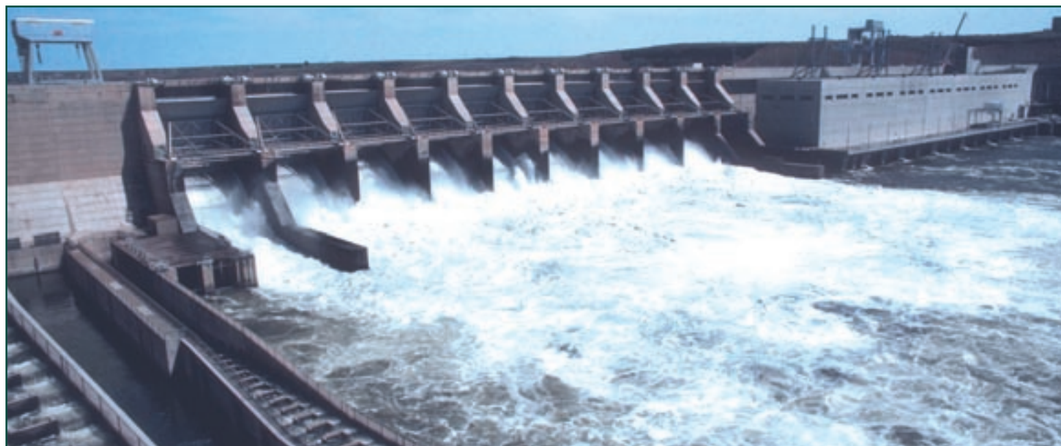
Ice Harbor Dam
