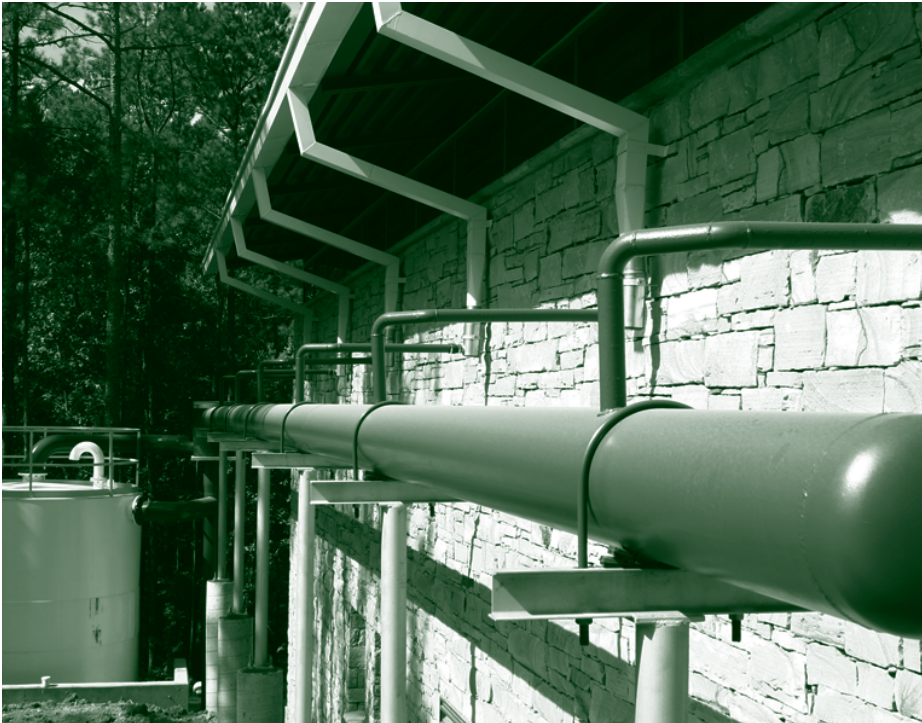
Water collected from the roof is reused as part of the building's sustainability practices.
