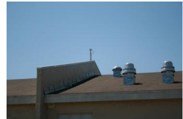
Figure 1. CORS GPS receiver mounted on top of a building in Courtland, AL.
