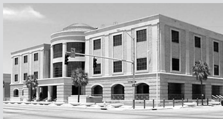
C. B. King Federal Courthouse Albany, Georgia
