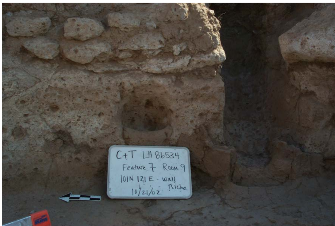
Figure 24.35. Room 9, masonry construction above bedrock.
