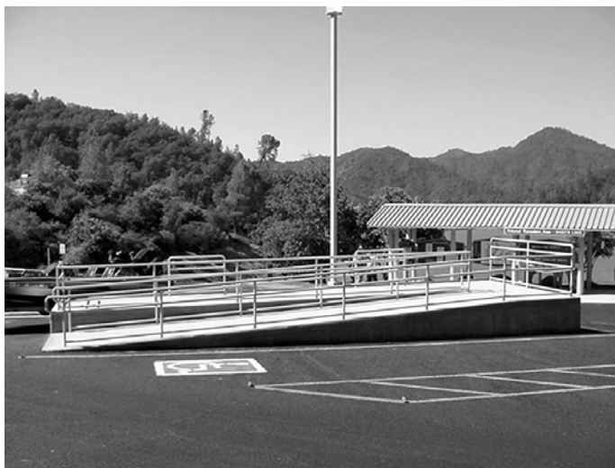
Accessible loading platform located at the Packers Bay public boat ramp at Shasta Lake.
