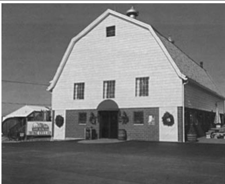
Shown above is a good example of how to reduce the risk of accidents in the parking area of a roadside market. This clean and smooth asphalt parking lot covers a large area near this winery shop and slopes gently up to the entrance, eliminating the need for steps. The entrance way is also well-maintained
