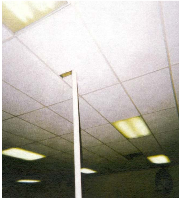
Ceiling Openings in SPD Work Room
