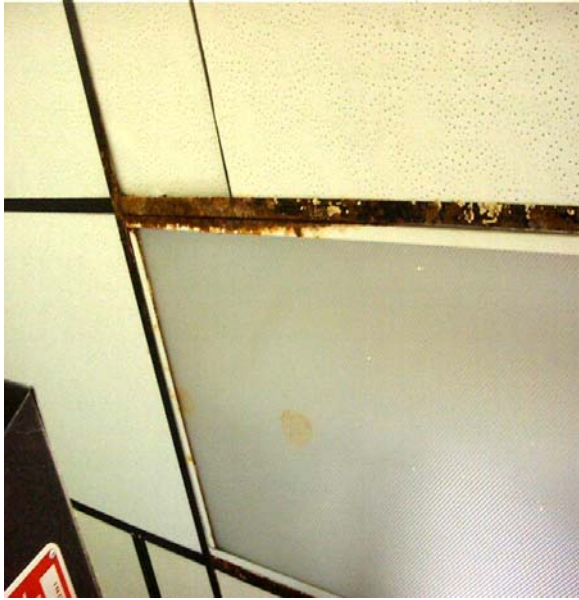
Corroding Ceiling Tile Struts in Orthotics Lab Dust on Window Sills in Cardiac Cath Lab
