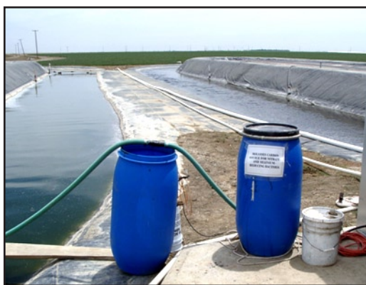
Figure 5 Molasses Injection for Carbon Source
