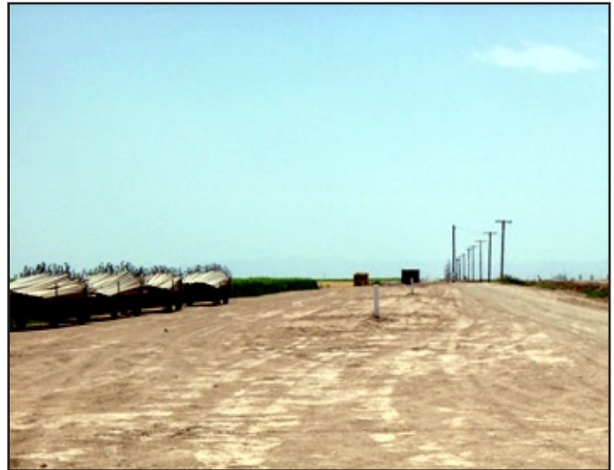
Figure 10 View Along Trench
