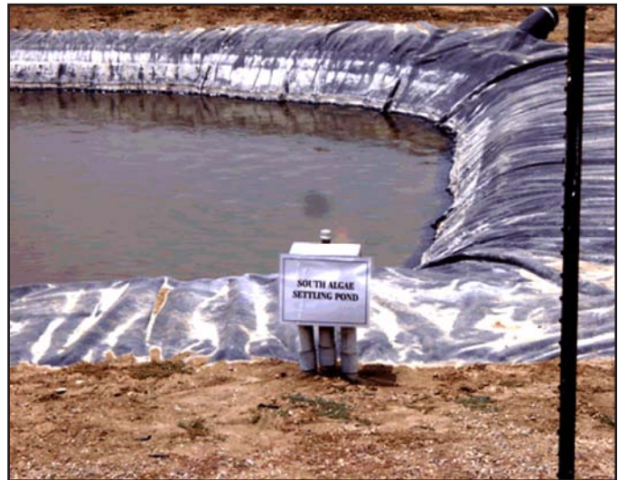
Figure 3 Deep Pond for Nitrate and Selenate Reduction
