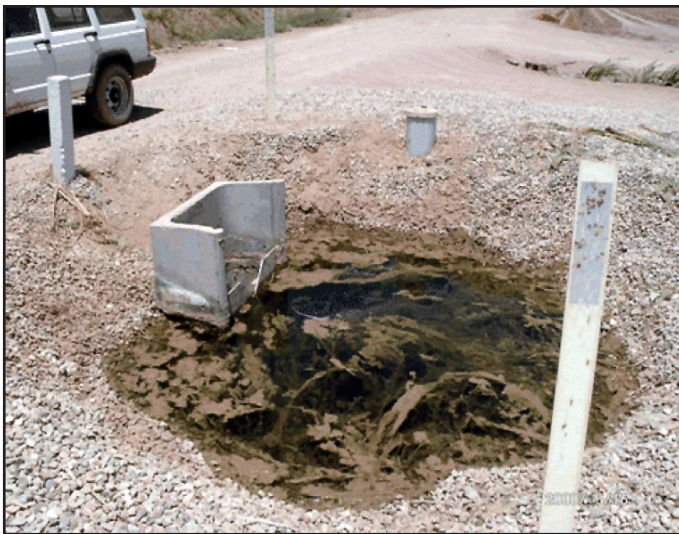
Figure 9 Outflow from Lewis Drain Treatment System
