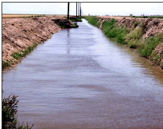
Figure 12 Widened Surface Drain with Gray Boards in Place
