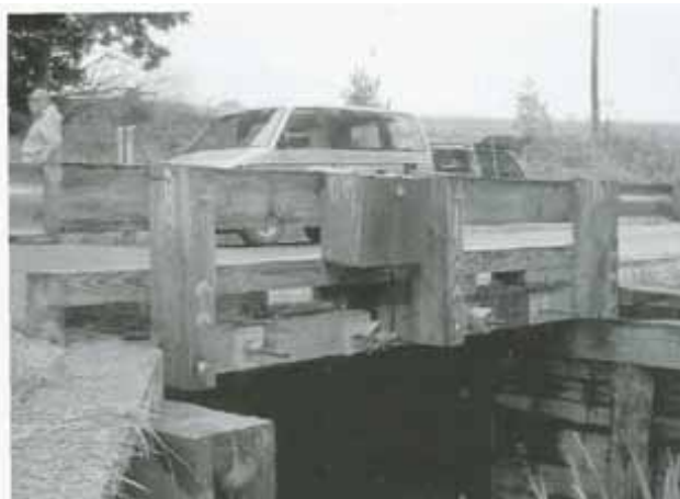
Figure 4.—McCurdy Road Bridge is ACQ treated.
