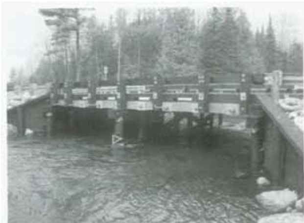
Figure 1.—Deck superstructure of the Graves Crossing Bridge is CCA treated.
