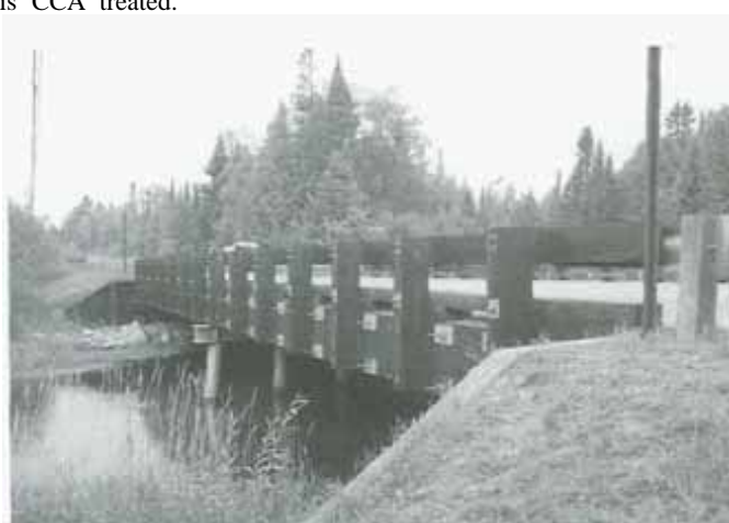
Figure 2.—Cameron Bridge is creosote treated.
