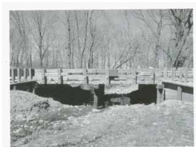
Figure 5.—Huntsman Road Bridge is ACQ treated with water-repellent additives.
