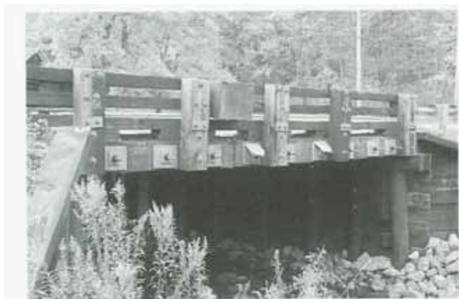
Figure 3.—Dutch Hill bad Bridge is creosote treated.
