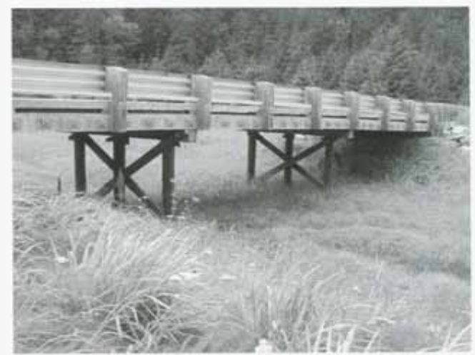
Figure 7.—Nelson Slough Bridge is naturally durable Alaska yellow cedar (untreated).
