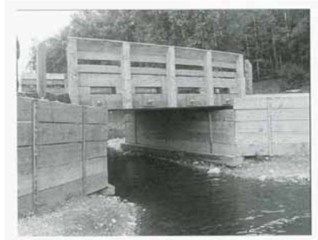
Figure 6.—Kepler-Bradley Bridge is copper fluoride treated.
