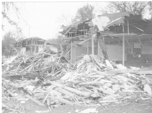
Waste generated at a building demolition project.
