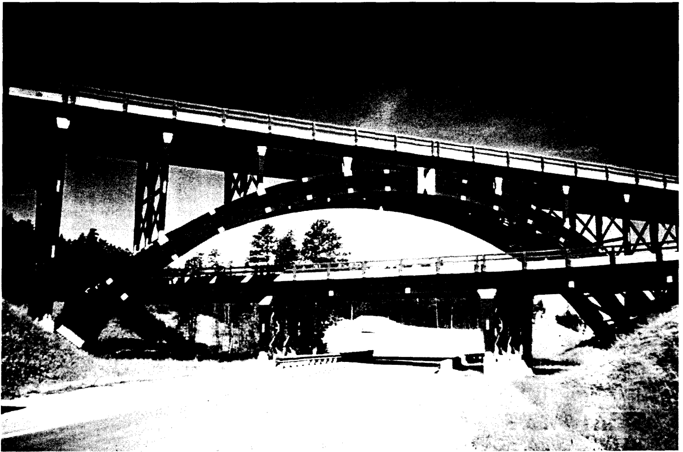
The Keystone Wye bridge, an arch bridge built with glulam beams (South Dakota), 1968.
