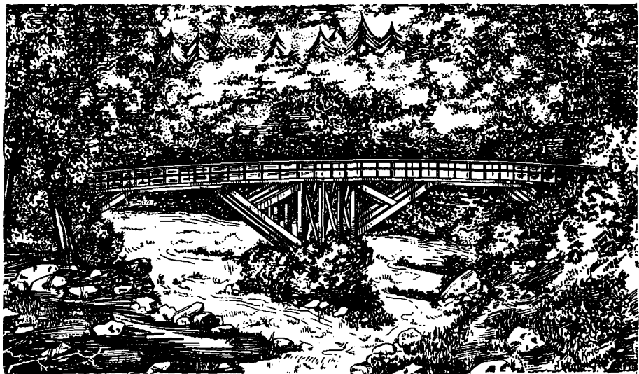
Enoch Hale's timber bridge over the Connecticut River (Bellows Falls, Vt.), 1785.
