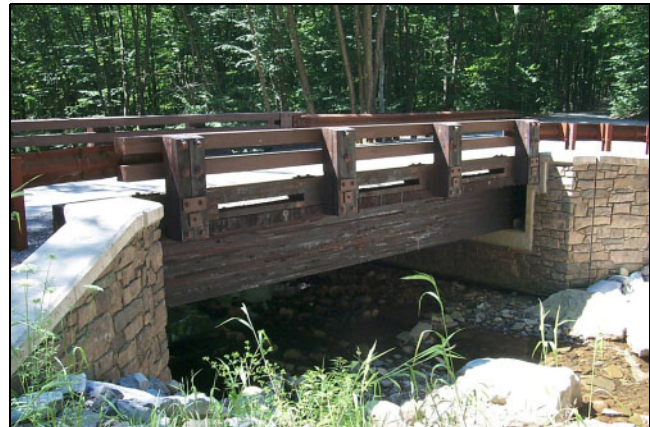
Glulam beams supporting the deck of a wooden bridge.
