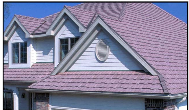
Roof shingles on FPL's research demonstration house are made from recycled plastic and wood fiber and are expected to last several decades.
