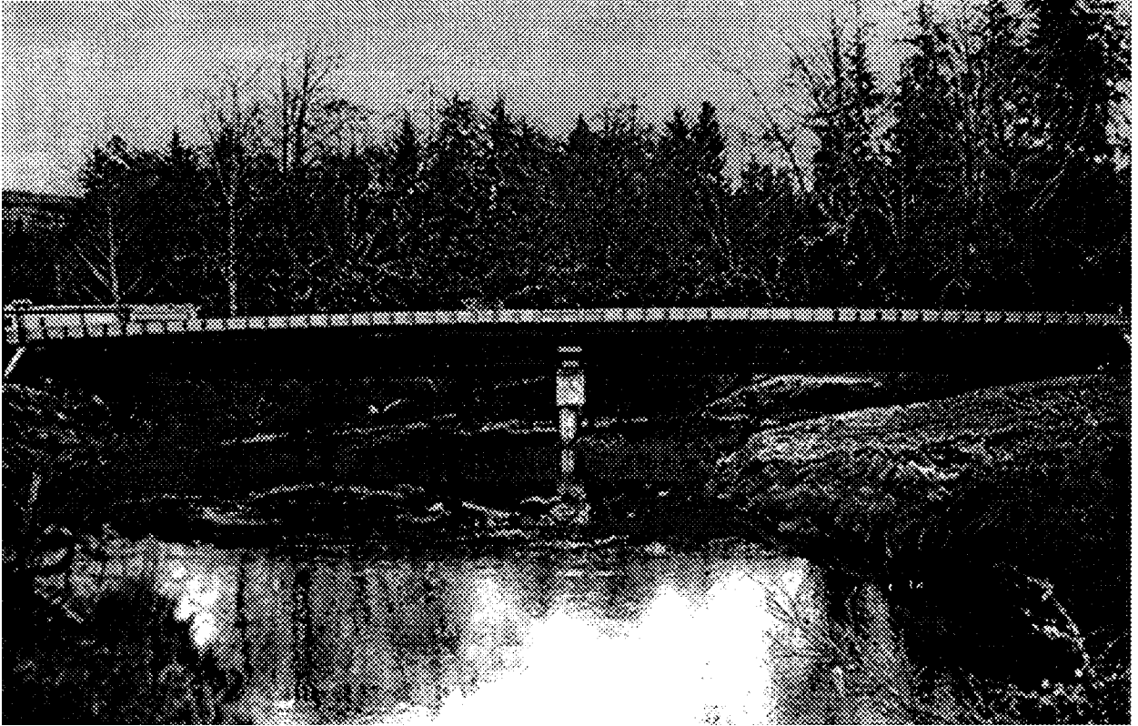
Figure 1-Side view of the Clallam Bay bridge.
