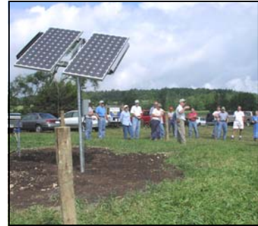
Solar panel for watering system
