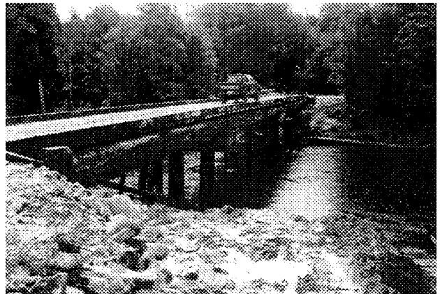
New Timber Stringer Bridge Savage River - Tasmania
