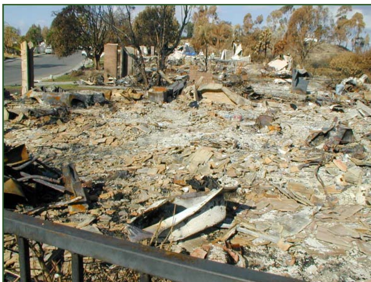
Fire damage to a housing subdivision in San Diego, California.
