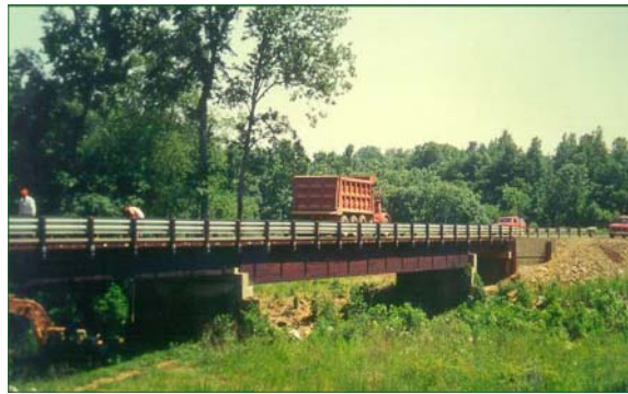
Glued laminated girder bridge.
