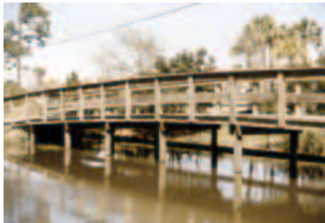
Figure 45—Fountains Bridge in Sandestin, Florida.
