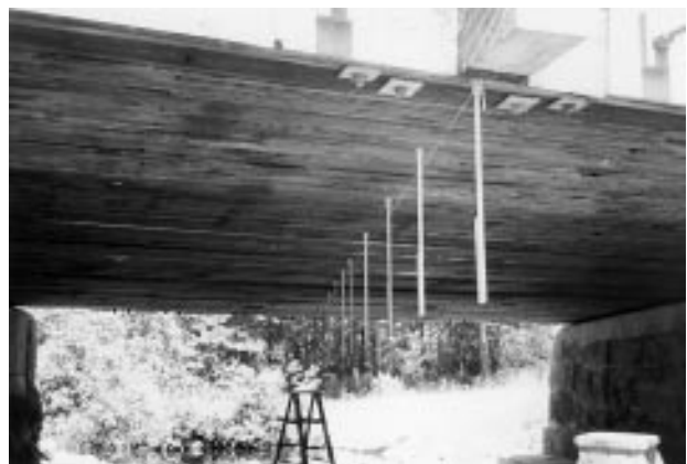
Figure 13—Load tests 1 and 2 (load test 2 shown) deflection measurements were obtained by reading values from calibrated rules suspended from the underside of the deck with a surveyor's level.
