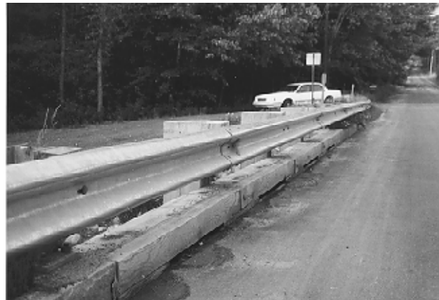
Figure 5—Completed Sanborn Brook bridge rail.
