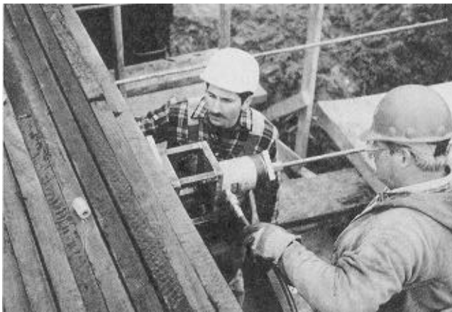
Figure 9—Bar tensioning bars using a single hydraulic jacking system.
