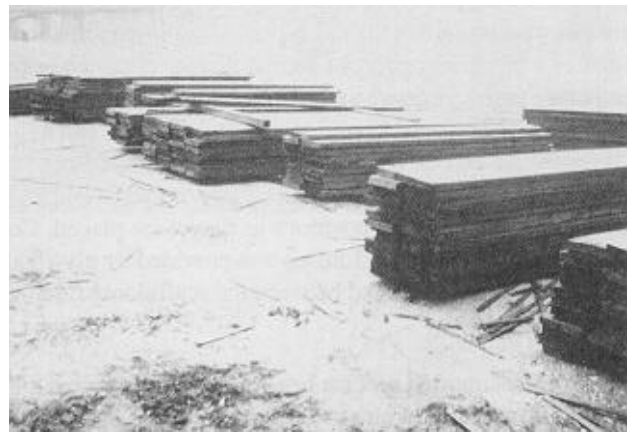
Figure 6—Eastern cottonwood laminations stacked at bridge site prior to construction.
