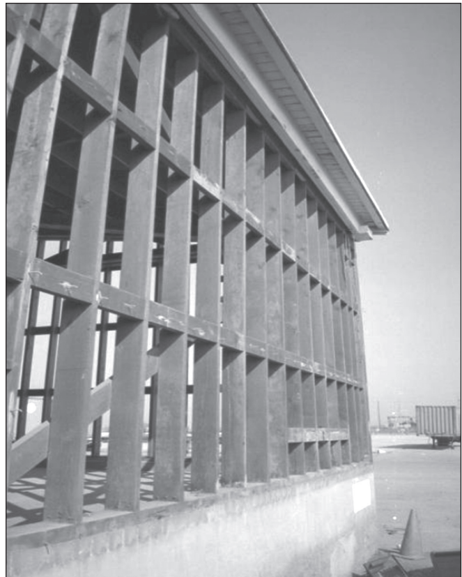
Figure 2—2 by 6 wall studs from the Naval Supply Center warehouse, Oakland, California.
