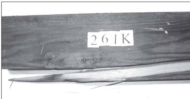
Figure 45—Example of toenail holes in an Oakland 2 by 6, potentially initiating a failure split.
