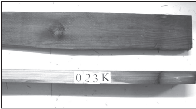
Figure 43—Example of failed 2 by 10 board where through splits from face nail holes caused horizontal shear failure.
