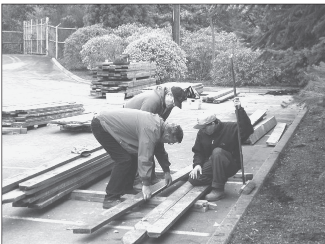
Figure 5—Crew grading lumber from University of Washington housing units, Seattle.
