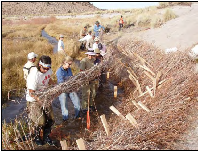
Class installing a brush mattress on Nov. 8, 2007 at Adobe Ranch near Bishop, CA
