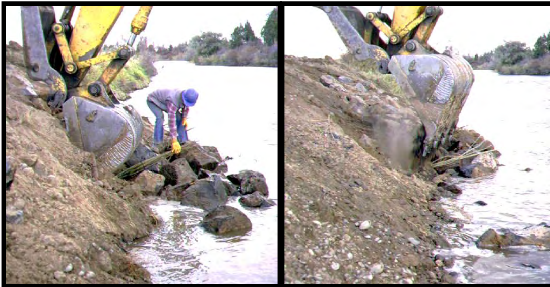
Figures 6 and 7: Excavator bucket is pushed into the streambank above the rock riprap in the keyway trench. Operator lifts the soil up (without pulling the bucket out) to create a small hole underneath. Another person shoves the willow bundle into the hole and the operator pulls the bucket straight out and the soil drops on to the bundle.
