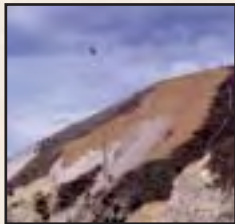
Road cut stabilization and restoration.
