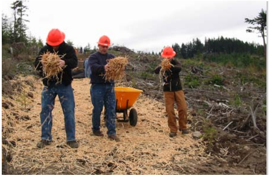
WOODSTRAW™ BEING APPLIED FOR EROSION CONTROL
