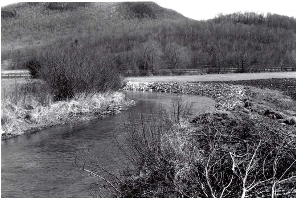
Figure 7.—Streambank stabilization along the Mettawee River protects this cropland from erosion and maintains the water quality of the river. The soil is Hero gravelly fine sandy loam, 0 to 3 percent slopes.
