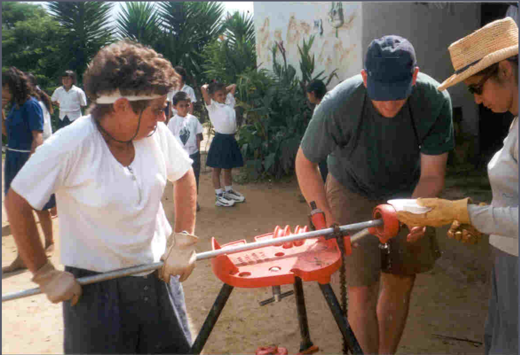
Pipe cutting and threading
