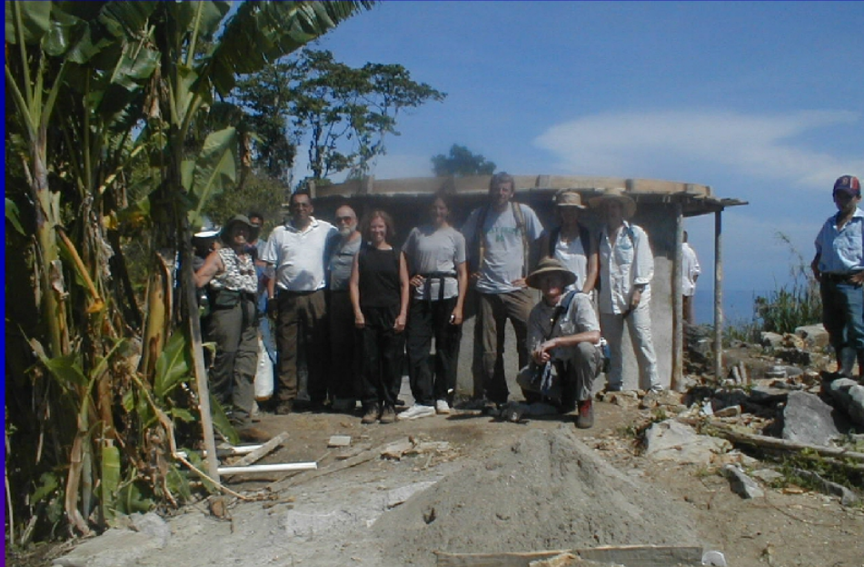
The water tank will look similar to this one at Nueva Vida
