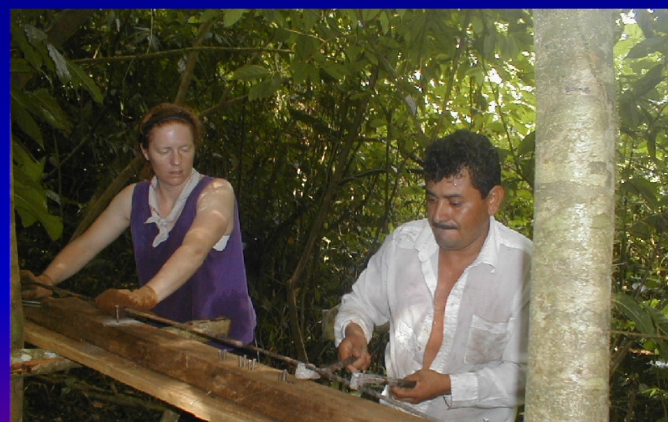
Cindy and Manuel (mason) building rebar reinforcement cages
