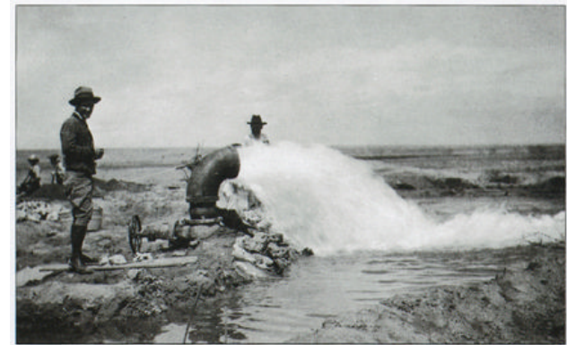
A.G. Fiedler, U.S. Geological Survey Figure 100. This flowing well was completed in the carbonate-rock aquifer 8 miles southeast of Roswell, N. Mex. On April 21, 1926, it flowed at a rate of 3,190 gallons per minute.
