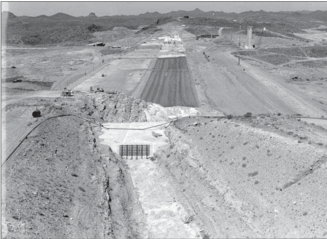
2.23. New Waddell Dam construction.
