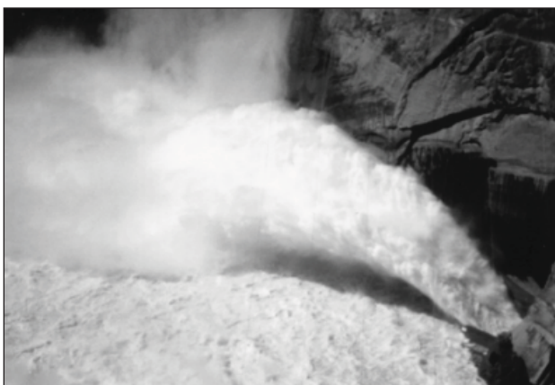
1.29. Basin X (tunnel flip bucket), spillway discharging approximately 27,000 ft 3 /s - Glen Canyon Dam, Arizona.
