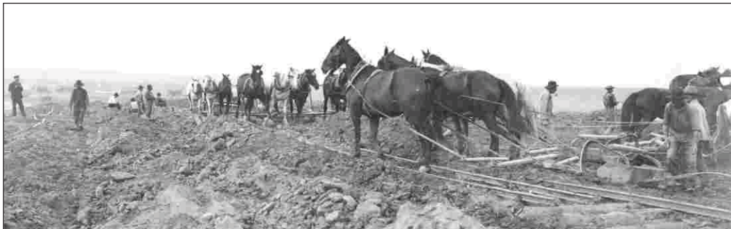
2.8. Belle Fourche Dam: Embankment fill construction.
