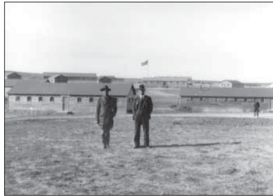
32.1. ECW winter camp at Belle Fourche Dam in 1934.
