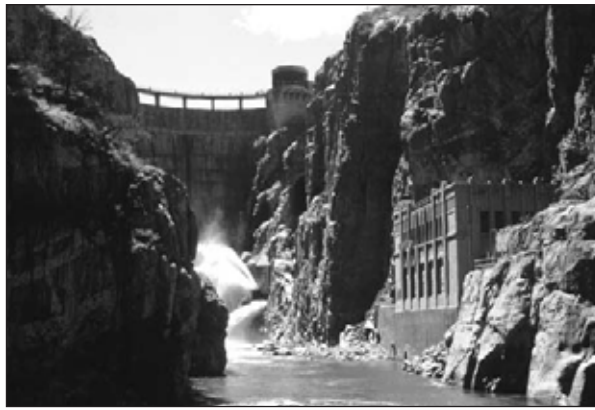
1.4. Buffalo Bill Dam (includes 1990 raised dam and replacement spillway), Wyoming
