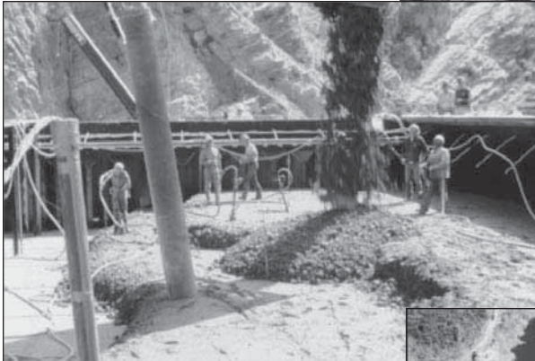
1.60. Placement and vibration of concrete in layers during modifications to Theodore Roosevelt Dam, Arizona.
