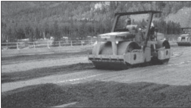
1.52. Compacting RCC at Stillwater Dam, Utah.
