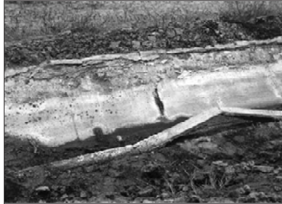
3.1. Concrete canal lining on the Central Valley Project.
