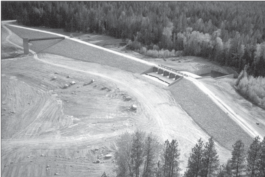
2.22. McDonald Dam: New dam in 2000.
