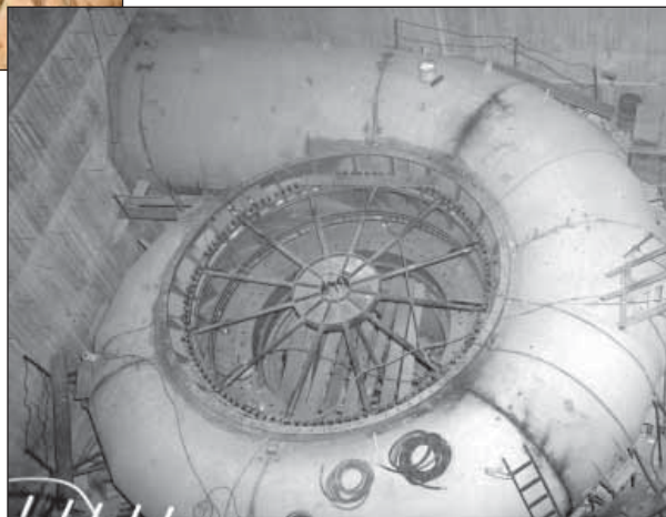
31.5. The scroll case in unit 5 of the Glen Canyon Powerhouse during installation in 1963.
