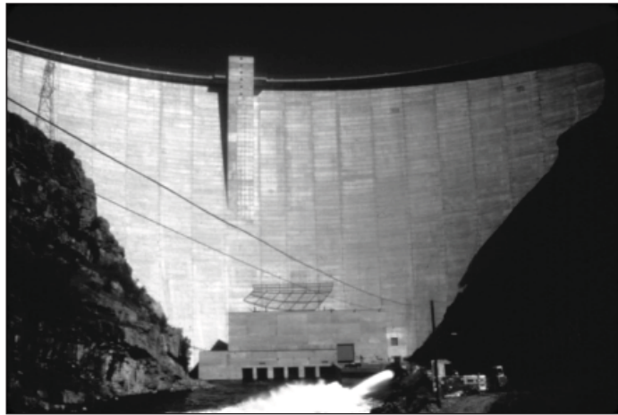
31.6. Flaming Gorge Dam and Powerplant in 1984.
