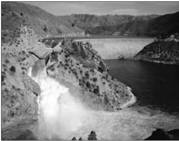
1.8. Arrowrock Dam, Idaho.
