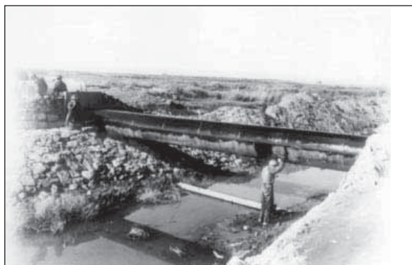
4.3. A CCC enrollee painting a pipe siphon across an open drain on the Gem Irrigation District, Owyhee Project, during February 1939.
