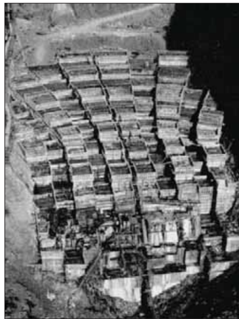
1.22. Hoover Dam, Arizona-Nevada. 50- by 50-foot concrete block placements
