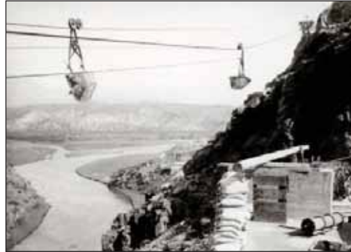
10.7. By 1907 the aerial tramway was delivering concrete from the batch plant to the Theodore Roosevelt Dam site. In order to reduce the cost of the project, Reclamation built a plant to manufacture cement at the dam site and even shipped cement down the Apache Trail to the construction at Granite Reef Diversion Dam.
