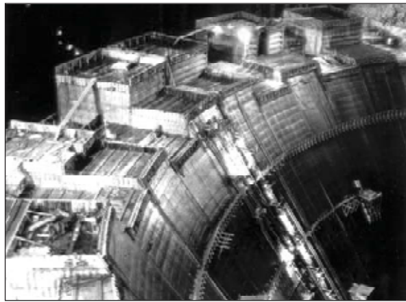
3.6. Block construction techniques reduced the potential for thermal cracking.
