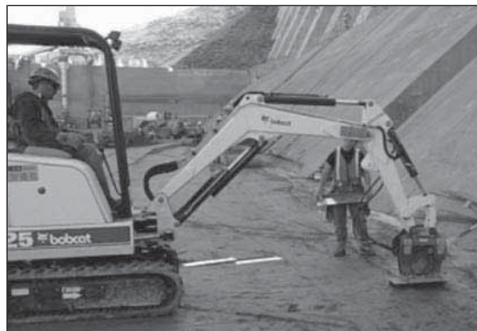
1.55. Installing joint inducing plates in RCC at Pueblo Dam, Colorado.
