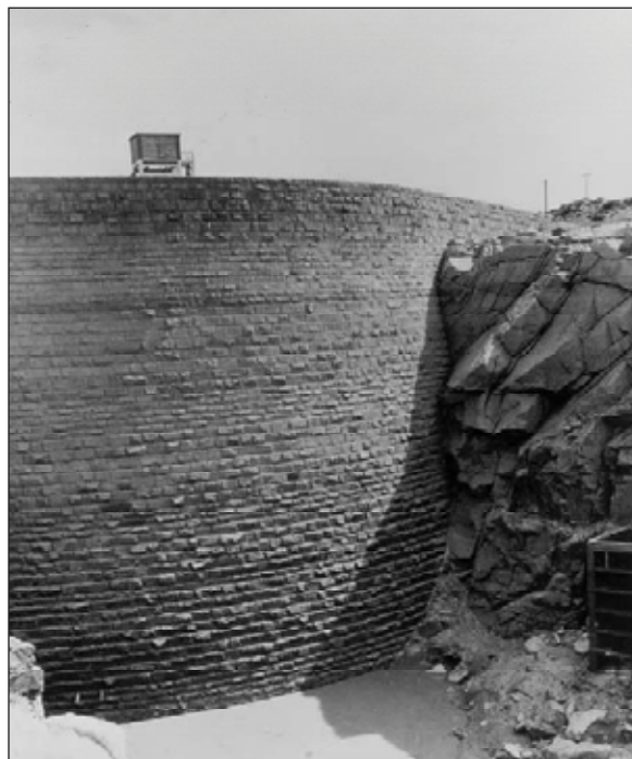
8.5. Upstream face of Pathfinder Dam on the North Platte River near Casper, Wyoming, is a masonry arch and cantilever section. Source: Bureau of Reclamation.
