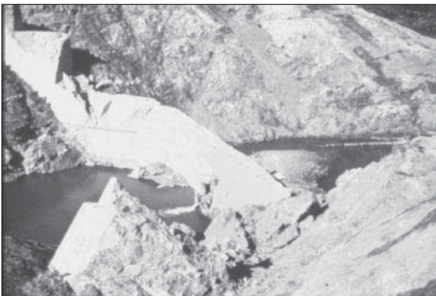
1.40. Malpasset Dam failure, Cannes District, France.
