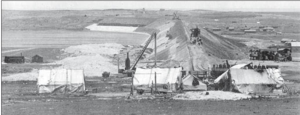
2.10. Belle Fourche Dam: Embankment from right abutment.
