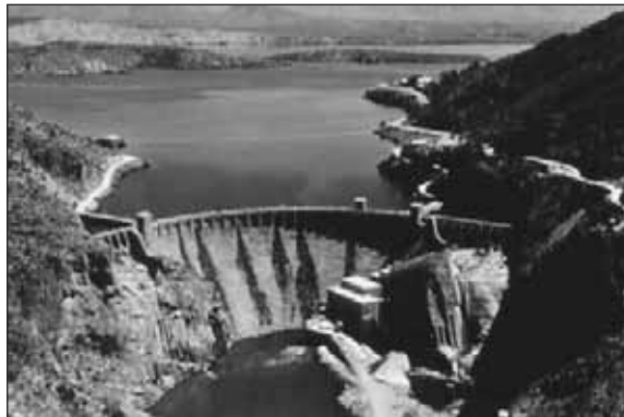
1.2. Original Theodore Roosevelt Dam, Arizona.
