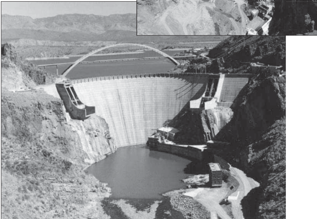
1.62. Modified Theodore Roosevelt Dam, Arizona, completed and rededicated in 1996.
