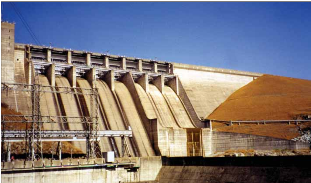
34.4. Folsom Dam spillway in 1998. The dam is a composite structure with a concrete spillway and earth wing dams on the American River above Sacramento, California. The U.S. Army Corps of Engineers built the dam between 1948 and 1956, but Reclamation manages the dam in cooperation with the Corps.
