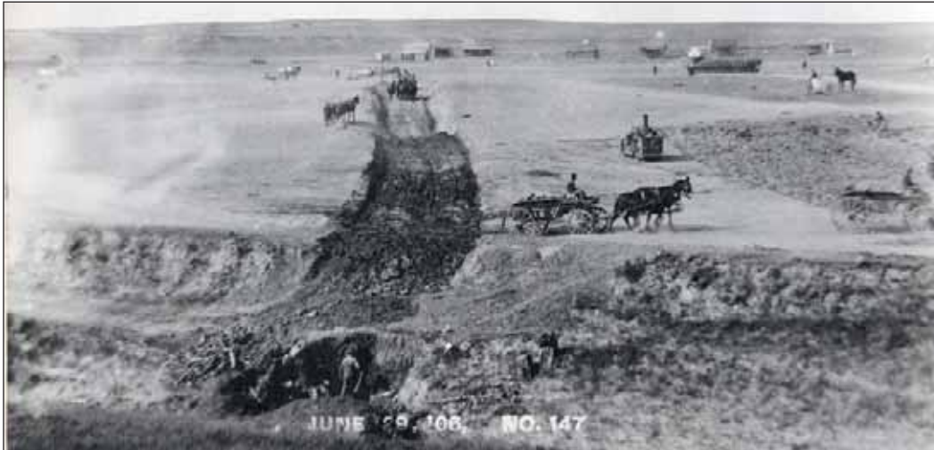
2.6. Belle Fourche Dam: Cutoff trench construction.
