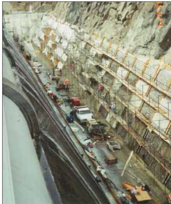
3.8. Tieton Dam spillway rehabilitated in 1999.
