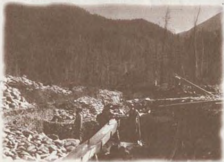
Figure 2. Sluice box operation on Lynx Creek. Gold-bearing gravel from the stream cut on the right of the photo was shoveled into the sluice box. ▼
