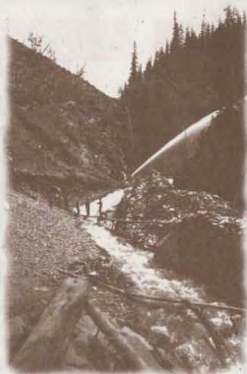
Figure 1. Hydraulic mining on Juneau Creek. Note hand-stacked boulders and precarious wheelbarrow bridge. ▶
