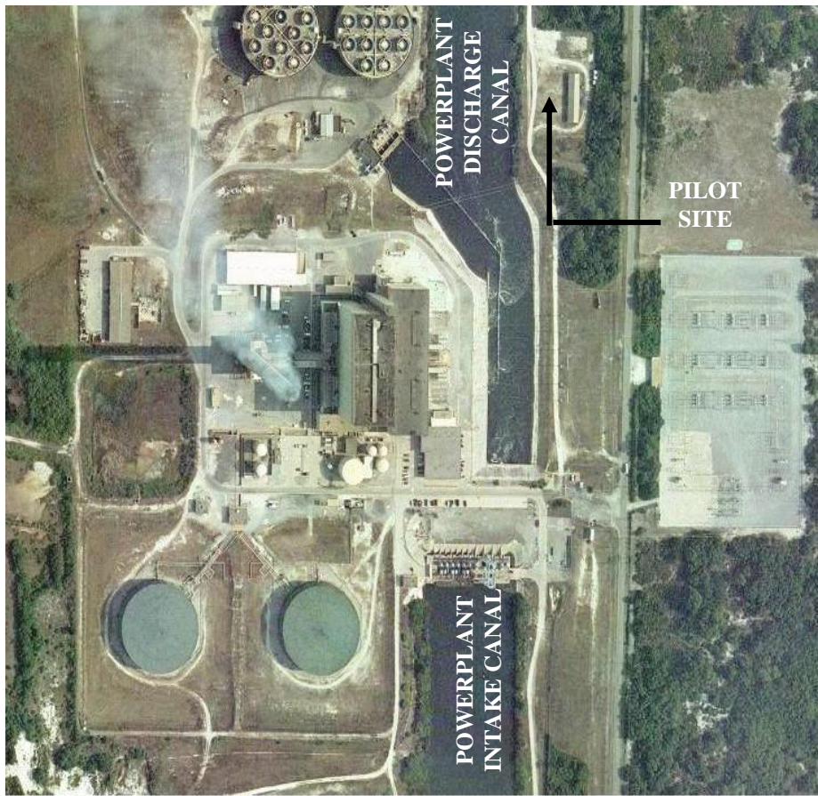
Figure 3-2. Aerial of the APGS and Pilot Testing Facility.
