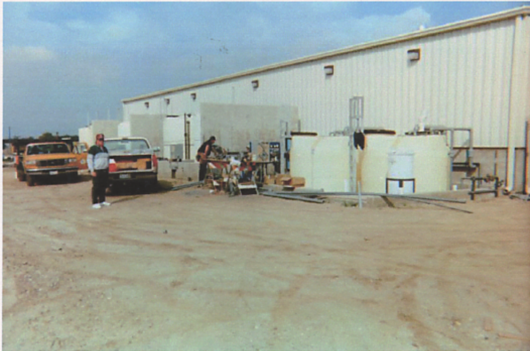
Figure 2.4. Chemical Storage Tanks Located behind Facility.
