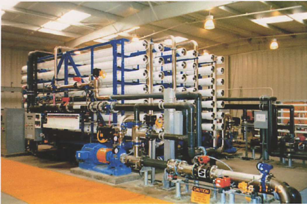
Figure 2.5. Reverse Osmosis and Nanofiltration Systems.
