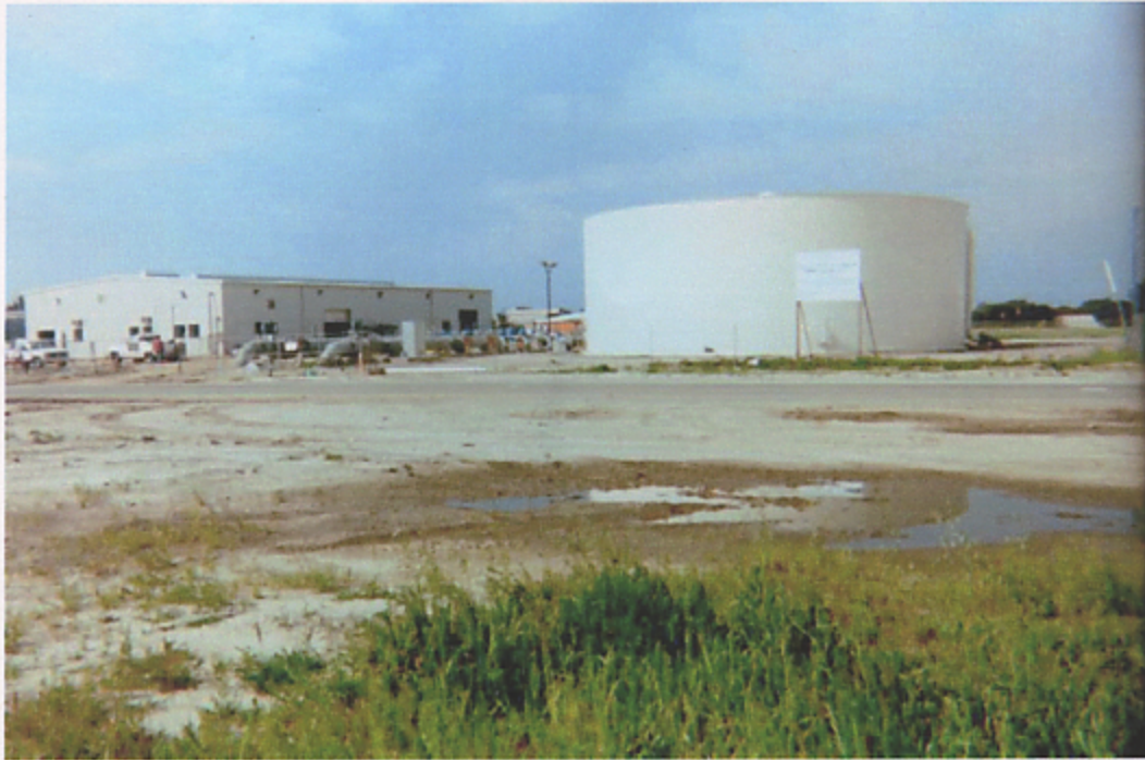
Figure 2.1. Port Hueneme Brackish Water Reclamation Demonstration Facility
