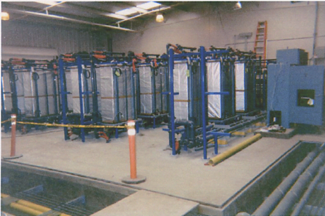
Figure 2.6. Electrodialysis Reversal System
