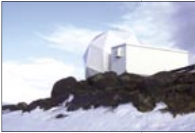
The Earth Station behind Palmer Station provides a communication link via the 5-meter-diameter antenna that sees a satellite orbiting the equator, allowing people to make phone calls and use the Internet, as well as providing the remote station with telemedicine capability.
