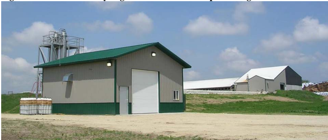
Figure 20 – Emerald Dairy Digester and Gas Cleanup Building
