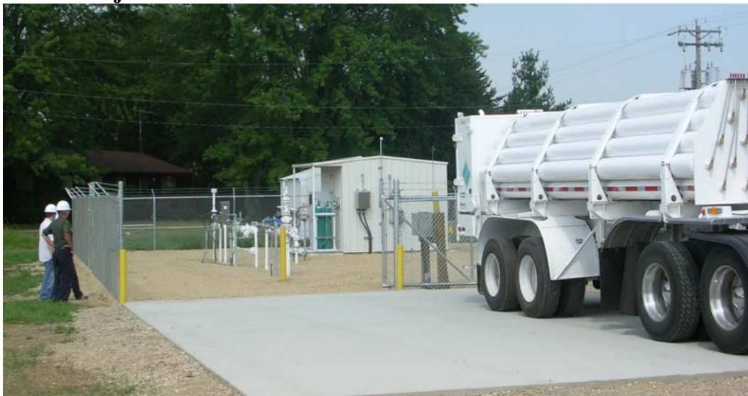
Figure 22 – Tube Tanker Truck at Injection Point
