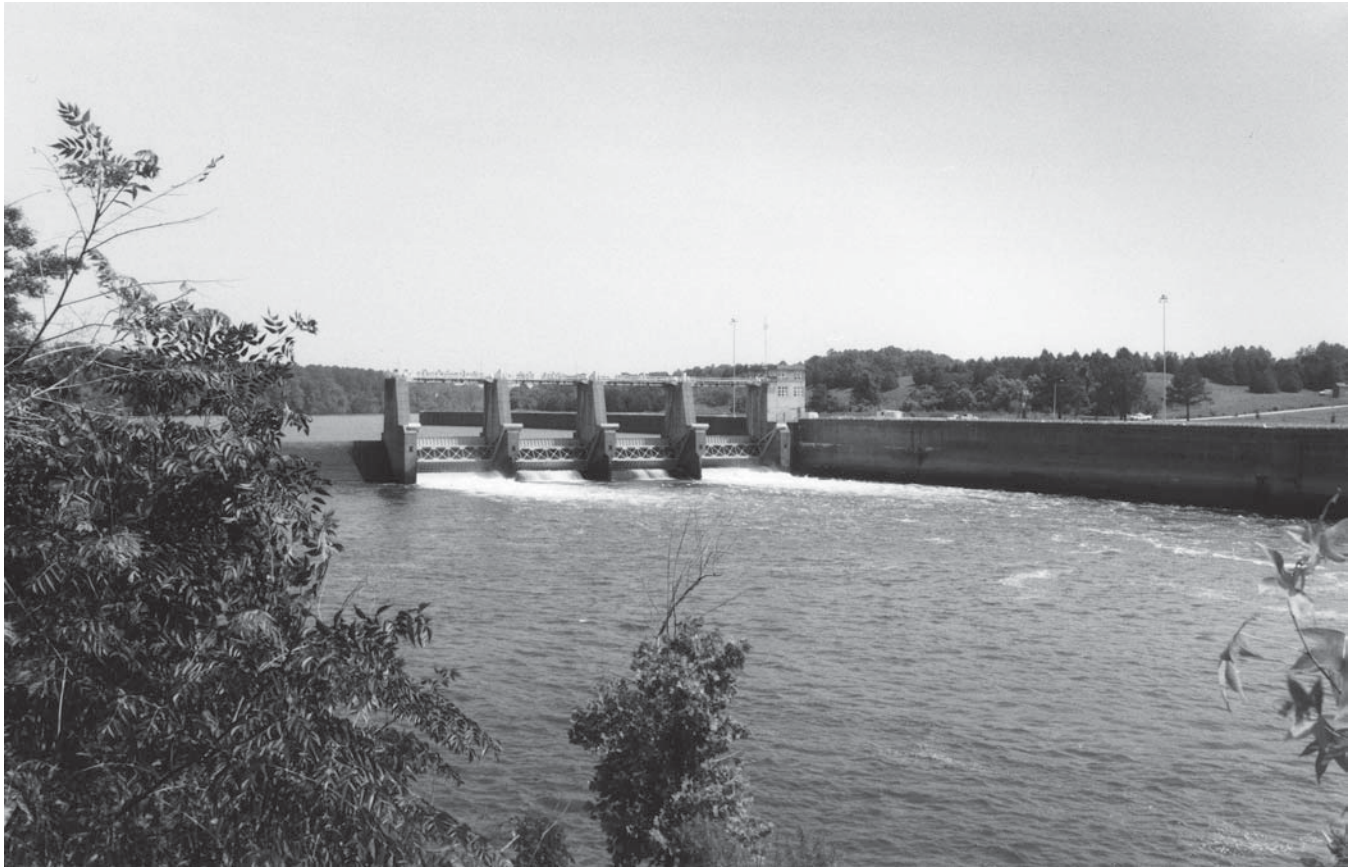
Figure 2.—Walter F. George Lock and Dam on the Chattahoochee River, which forms the eastern border of Houston County. The soils on the flood plains along the river include Annemaine, Kenansville, Kolomoki, and Riverview soils.
