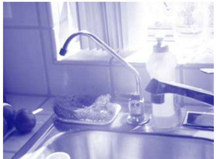
Figure 1: Treated water from reverse osmosis units is usually dispensed from a separate faucet (1).
