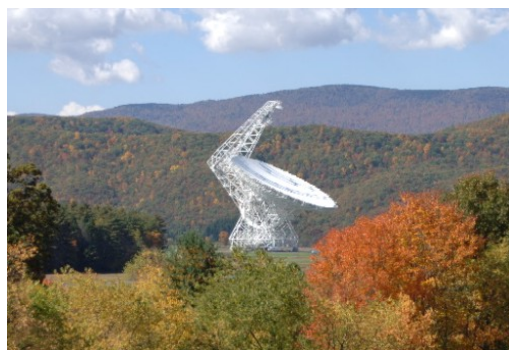
The Green Bank Telescope (GBT) in West Virginia is the world's largest, fully steerable radio telescope. Described as a 100-meter telescope, the actual dimensions of the surface are 100 by 110 meters. The overall structure of the GBT is a wheel-and-track design that allows the telescope to view the entire sky above 5 degrees elevation. The track is level to within a few thousandths of an inch in order to provide precise pointing of the structure while bearing 7,300 metric tons of moving weight. Credit: NRAO/AUI/NSF
