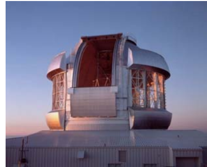
Gemini North dome/enclosure with setting sun (to left) lighting up bottom half of telescope through thermal vents (fully open). The observing slit is partially open revealing the truss and top end of the telescope. Credit: Neelon Crawford, Polar Fine Art; Gemini Observatory/AURA and NSF
