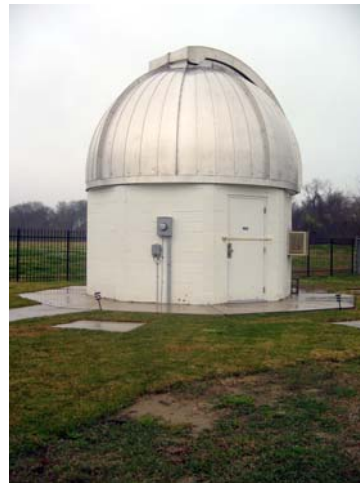
Observatory just adjacent to the brown-field site -City of Gretna
