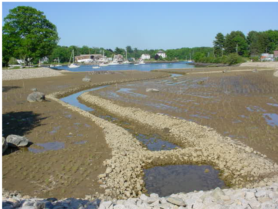
Salt Marsh Establishment After Consolidation and Backfilling
