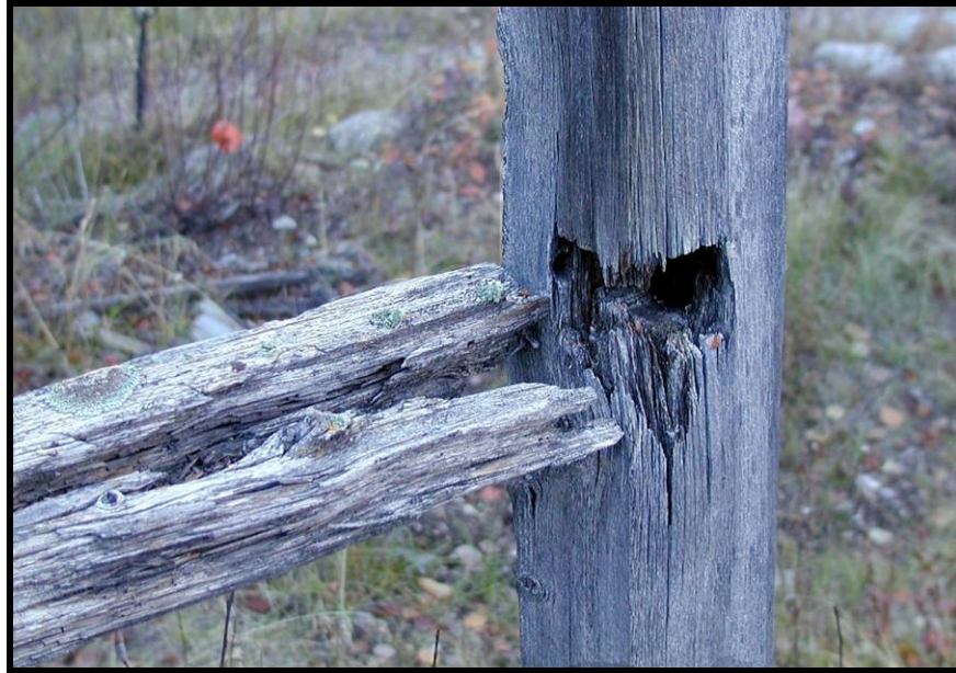
Figure 20. A grave enclosure corner post with signs of internal decay.
