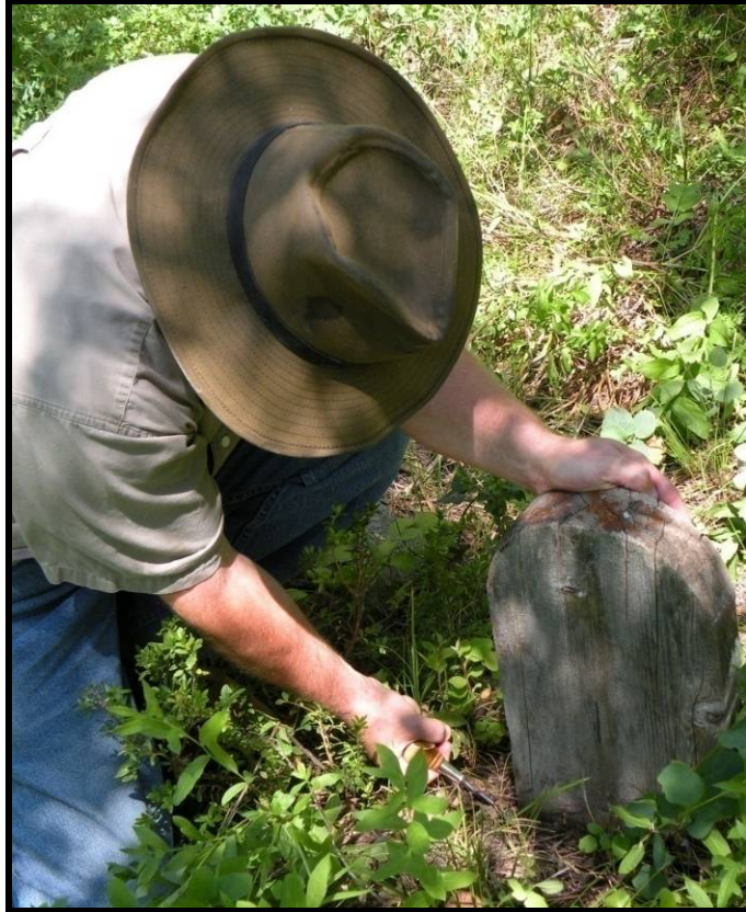
Figure 33. Probing at the base of a marker with an awl to check for deterioration.
