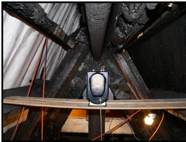
Figure 107. Source placement for digital radiography at Location A on Truss 7.
