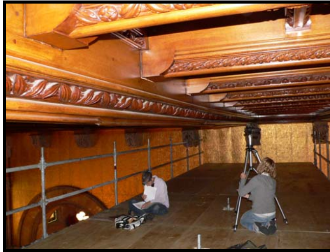
Figure 109. Scaffolding platform used for radioscopy setup.
