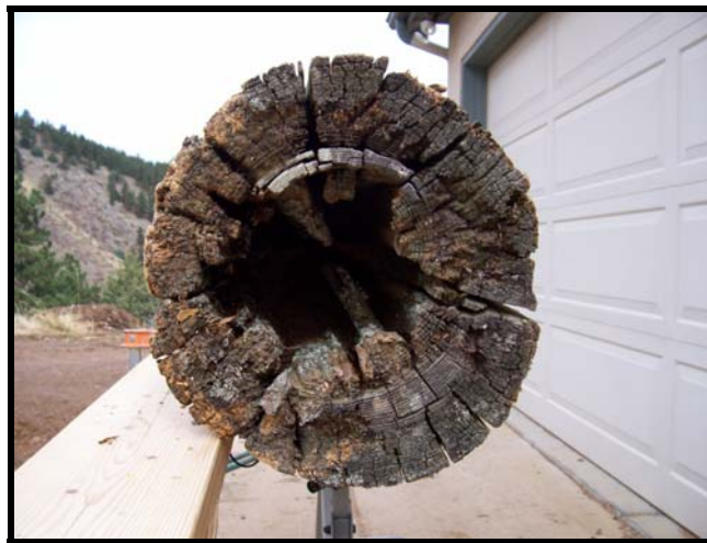
Figure 49. Decayed log section.
