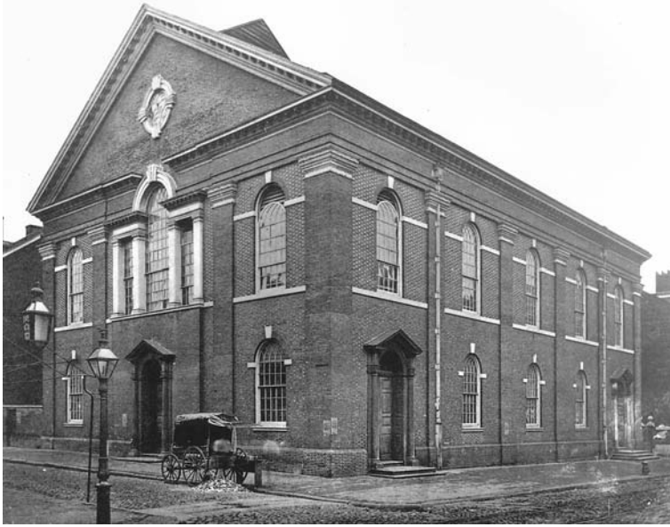
Fig. 6. Zion Lutheran Church, Fourth and Cherry Streets, Philadelphia, 1766-69, photographed ca. 1869. Robert Smith's handsome brick exterior walls survived a 1794 fire, allowing the church to be rebuilt within them. Author's collection.
