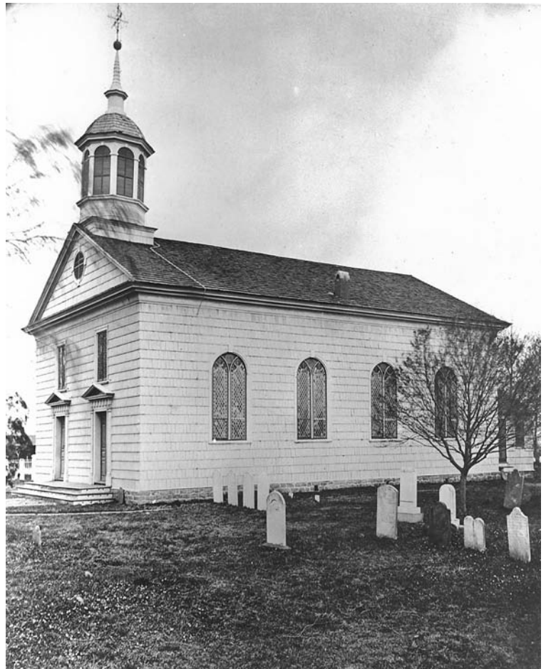
Fig. 9. Christ Episcopal Church, Shrewsbury, N.J., 1769-74, photographed ca. 1870. Secondhand stained glass had been installed in the original window openings in 1867, but other elements of the exterior remained essentially unchanged until the addition of a tower in 1874. The building is framed in oak and shingled in white cedar. Photo courtesy of Christ Episcopal Church.
