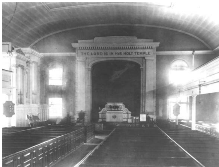
Figs. 4 and 5. St. Paul's Episcopal Church, Third Street, Philadelphia, 1760-61. Interior view below, ca. 1900, shows its appearance following renovations of 1830 and later. The graceful arched ceiling shows the effect possible under a raised bottom chord truss. Ceiling framing can also be seen in the pattern of staining on the plaster surface. At 65 ft. clear span, St. Paul's represented Robert Smith's widest use of the raised bottom chord truss. Photos courtesy of Episcopal Community Services.
