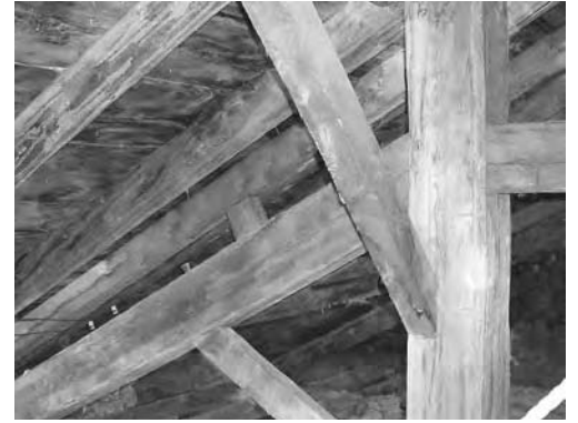
FIG. 12. DETAIL OF TOWER TRUSS, UNITED CHURCH, CRAFTSBURY, VT., 1816.
