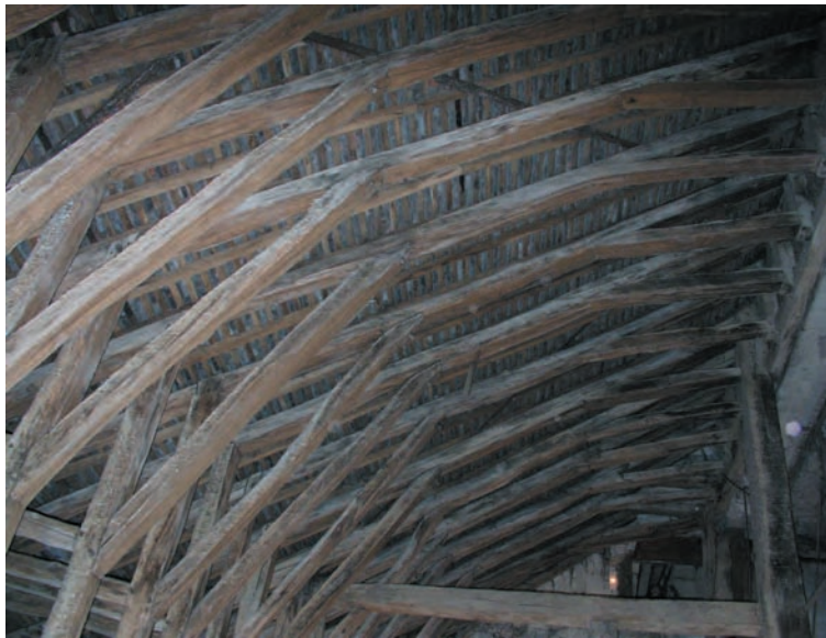
Roof framing at Ste. Madeleine, Troyes, 12th century.
