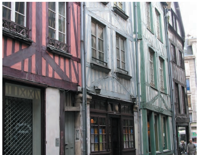
At top, in Rouen, a charnel house in the era of the Black Death, now put to use as an art school. Above, shopfronts with trussed breast beams over the openings. The braces are termed "décharges couplées."
