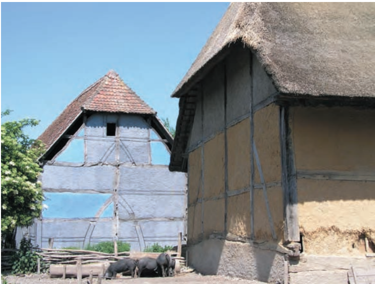
Parti-colored wattle-and-daubed barns at the Ecomusée d'Alsace, with outlined timbers. Note typical jerkin-head roof, with truncated ridge to allow a short hip that gives some protection to the gable end.
