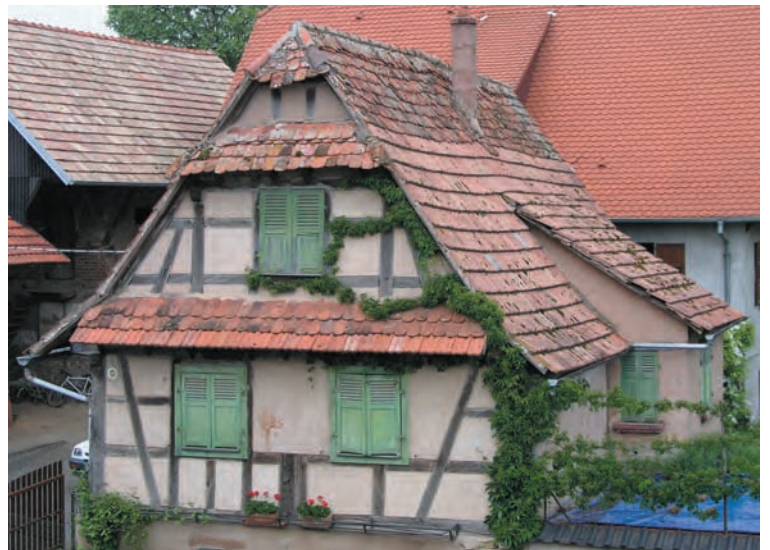
Small traditional Alsace house, half timbered, with tiled, jerkin-head gable roof and pentices over the gable windows, at the Ecomusée d'Alsace in Ungersheim.
