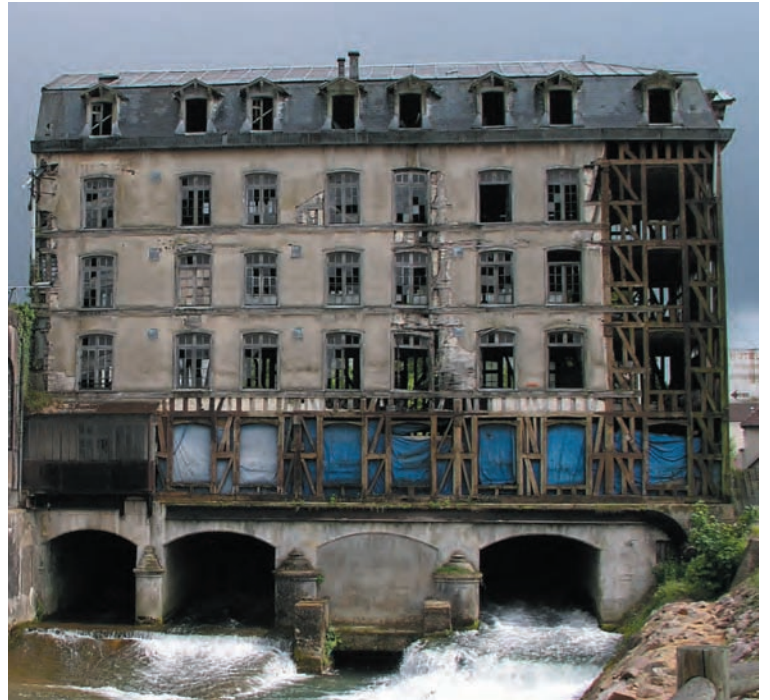
Five-story derelict 19th-century water-powered mill, Bar-sur-Seine. Heavily framed, originally infilled and stuccoed and with a Mansard slate roof; it awaits an angel or a recycler. Detail below.
