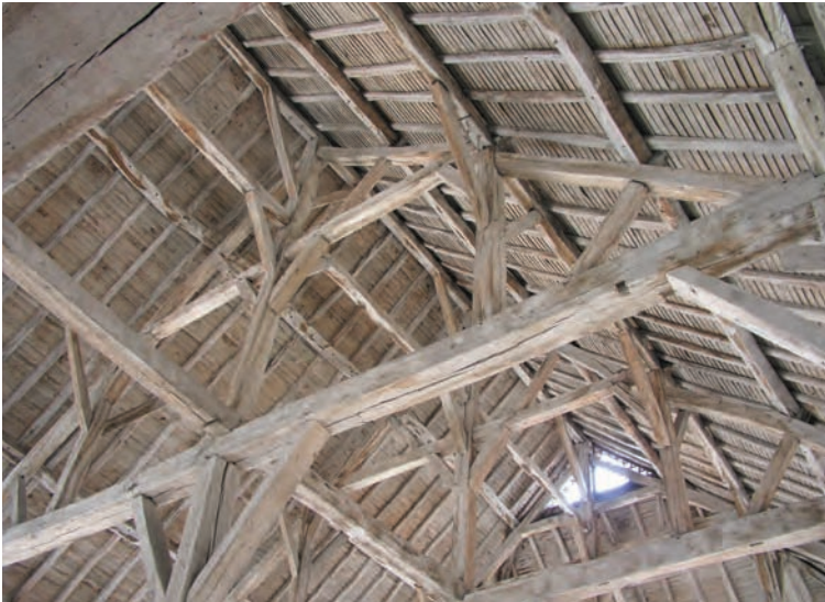
Hipped roof of the 16th-century market hall (restored) at Piney, in the Champagne region. At right above, detail of necked tying joint, in which the tie beam is bridled over the post top and a twin tenon projects up from the latter to enter the underside of the plate.
