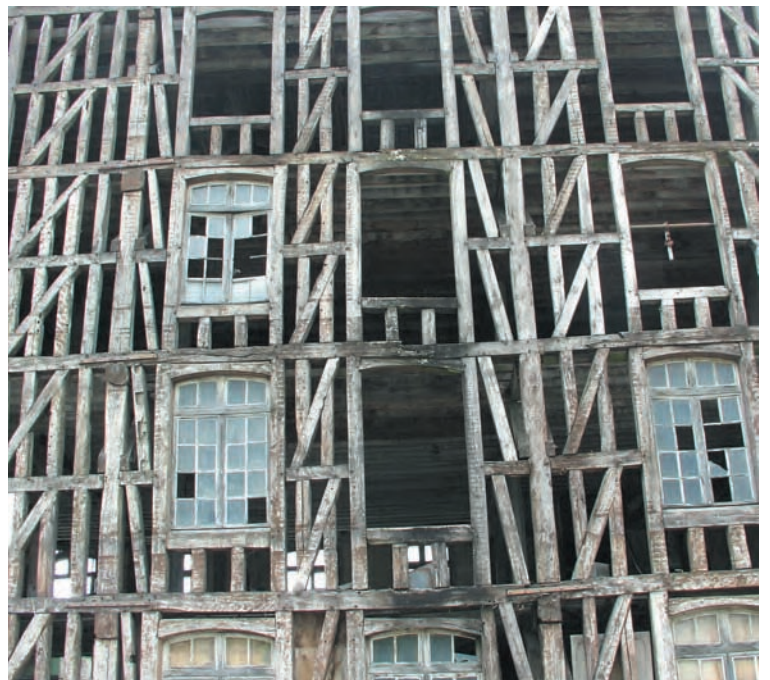
Five-story derelict 19th-century water-powered mill, Bar-sur-Seine. Heavily framed, originally infilled and stuccoed and with a Mansard slate roof; it awaits an angel or a recycler. Detail below.
