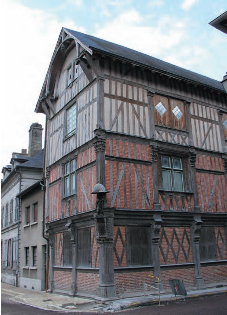
Conspicuous 16th-century house at Bar-sur-Seine, with remarkable carved frame, framed gable-end overhang, brick and stucco infill. There seems to be a municipal problem at the corner.
