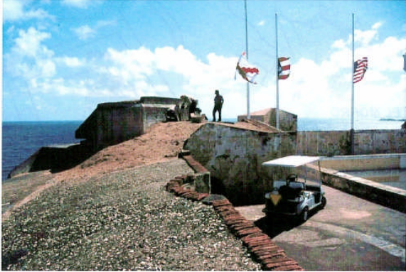
Figure 6: Roofs of the rooms (casemates) on the north edge of the Plaza de Armas in El Morro were filled with dirt to provide protection against shell bombardments from enemy ships approaching from the Atlantic Ocean. Several pieces of wood with apparent termite damage were found on top of the roofs, and activity of C. havilandi (MORO2) and Heterotermes sp. (MORO3) were detected by stake survey.
