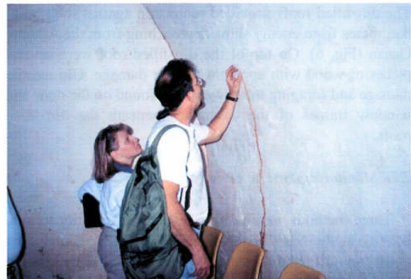
Figure 5: Extensive foraging tubes of C. havilandi were found on the walls and floors of Casemate 19 facing the Plaza de Armas in El Morro.
