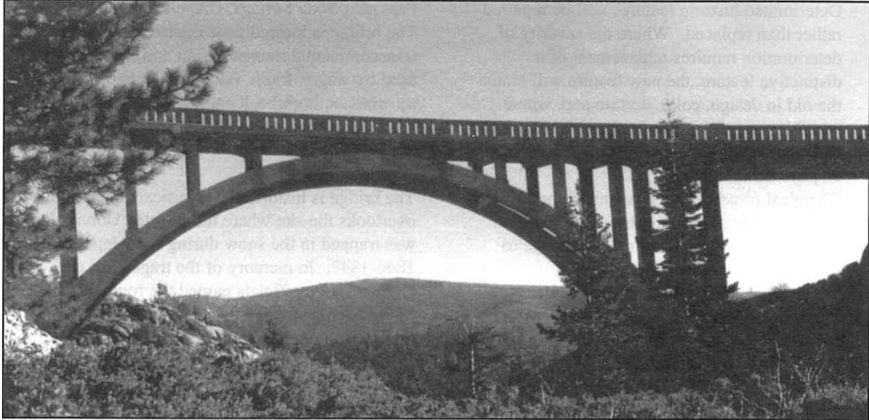
Rehabilitated Donner Summit Bridge. (October 1995)
