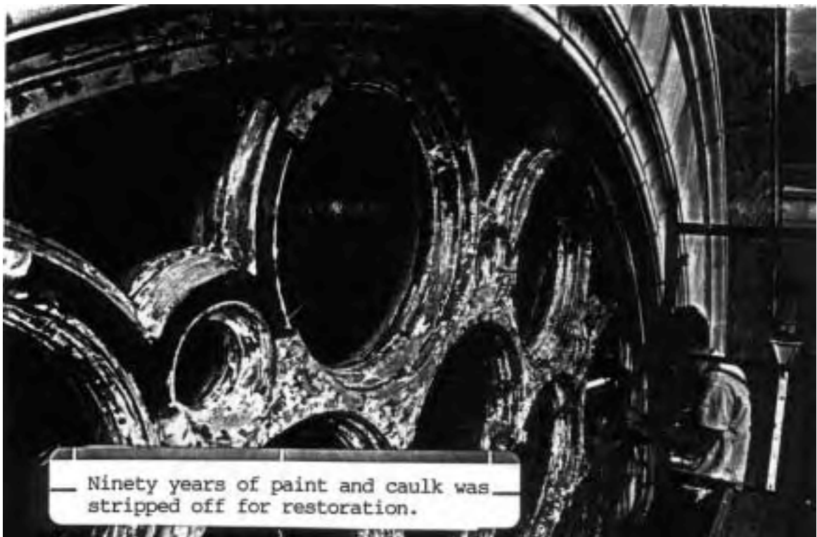
All the stained glass was removed to restore the frame.
