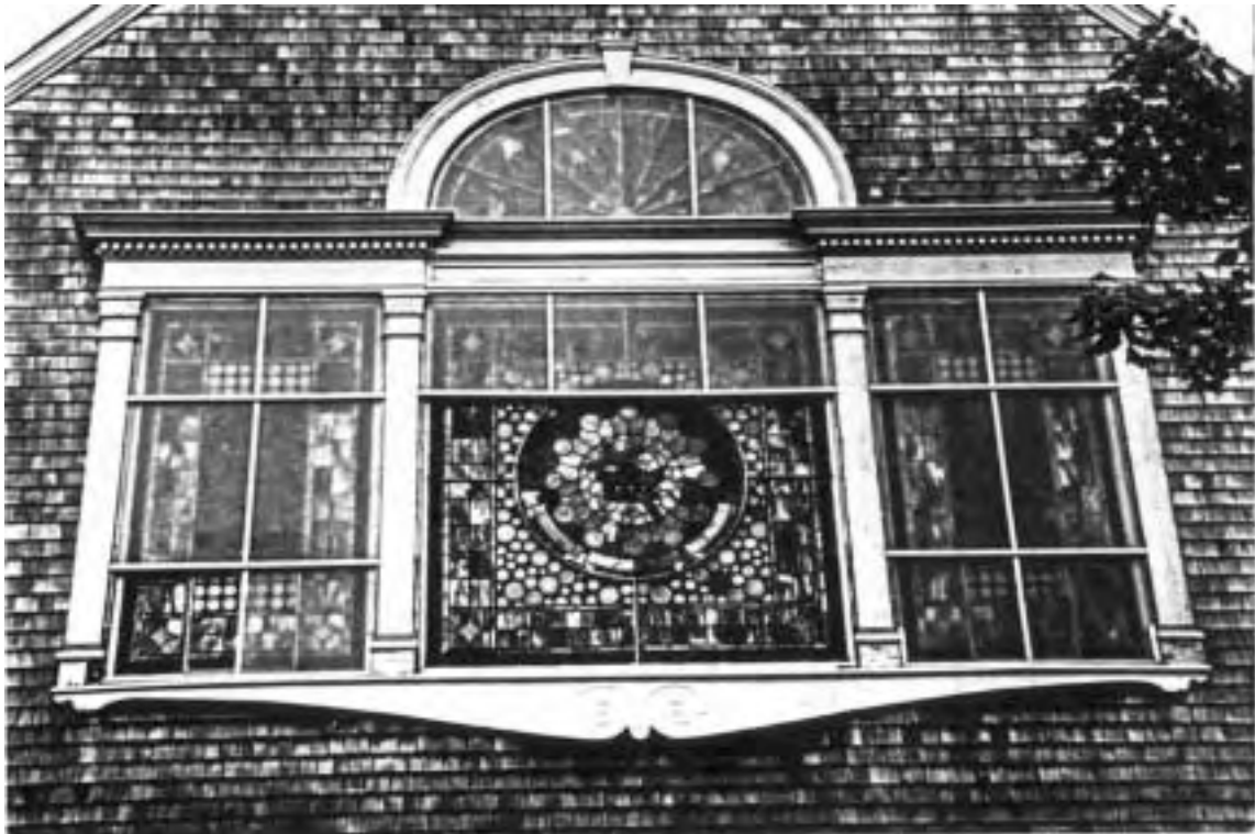
—Removal of the hazed PG revealed the --brightly colored class behind.
