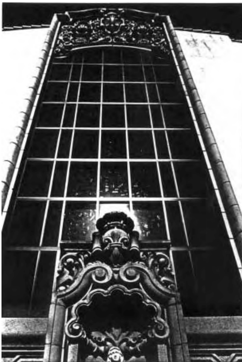
Fig 16. PG was installed over slab glass in 1993 on this church in Phoenix, AZ.
