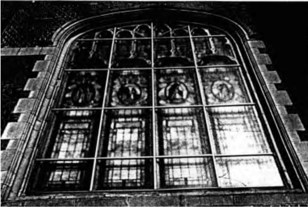
Fig 27. The art glass in this installation is blurred by glare and textured PG.
