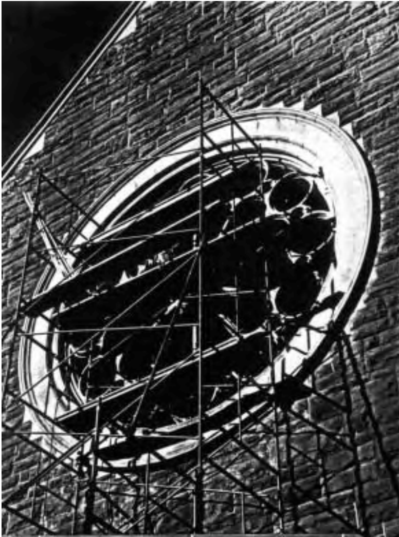
All the stained glass was removed to restore the frame.
