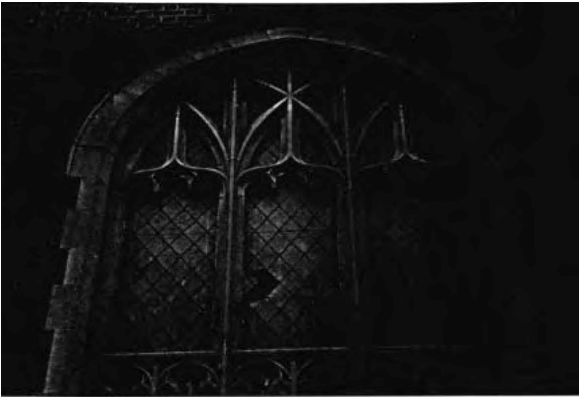
Fig 11. 1922 diamond-pane windows became PG for stained glass installed later.
