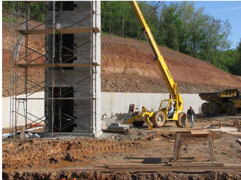
Fire Station under construction – April 2008.
